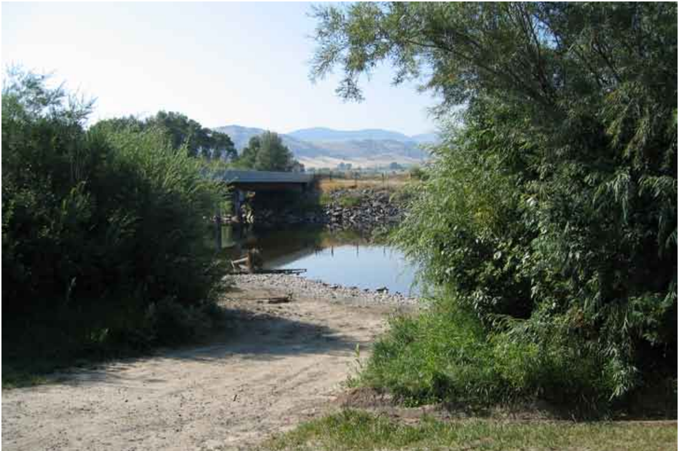
Mayflower Bridge FAS - Jefferson River near Whitehall
